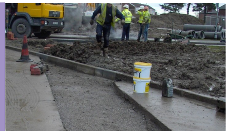
Concreting of Gough Road
