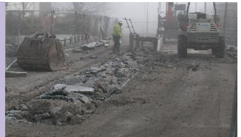
Excavation of Gough Road
