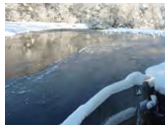
Inlet from River Swale
